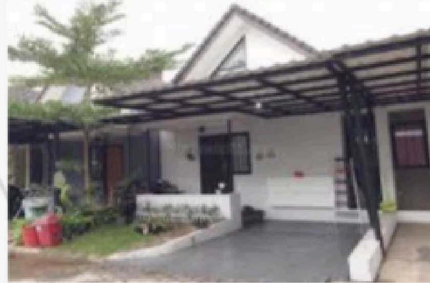
Habitat Terrace Residence Serpong
